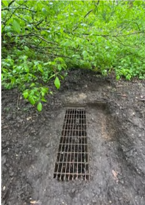
Grate near Frog Pool, cleared by volunteer "Sam" Samuels
